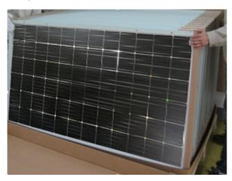
1.3.7 Move the modules. Two people hold the two short edge of the module, while the strength, the module to the designated location. Wear protective gloves during unpacking to avoid scratching your hands. Please grab the inner side of the frame to move the modules. Do not let your fingers touch the glass surface. Avoid leaving fingerprints on the glass surface.
