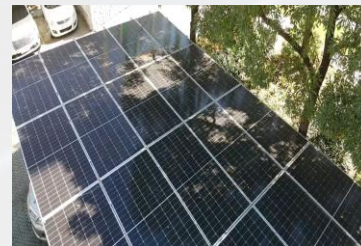
Shade from trees in carport environments, long-term impact on string power.
