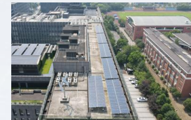
Rooftop Plant @Zhejiang 5.5% increase in lifecycle energy yield due to no shading.
