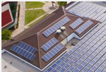
Avoid installation in shaded areas, low utilization of rooftop space.
